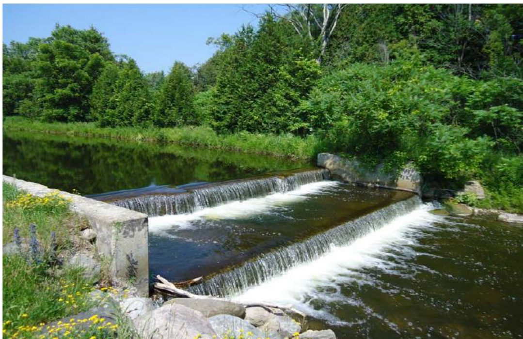
Figure 4.2-1: Photo of Warkworth WTP Looking Upstream
