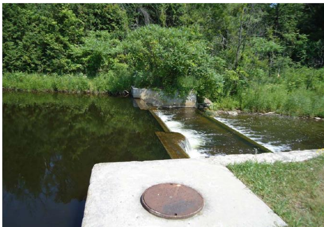
Figure 4.2-2: Photo of Warkworth WTP and Manhole
