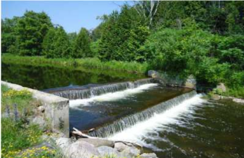
Figure 4.2-1: Photo of Warkworth WTP Looking Upstream
