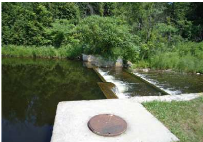
Figure 4.2-2: Photo of Warkworth WTP and Manhole
